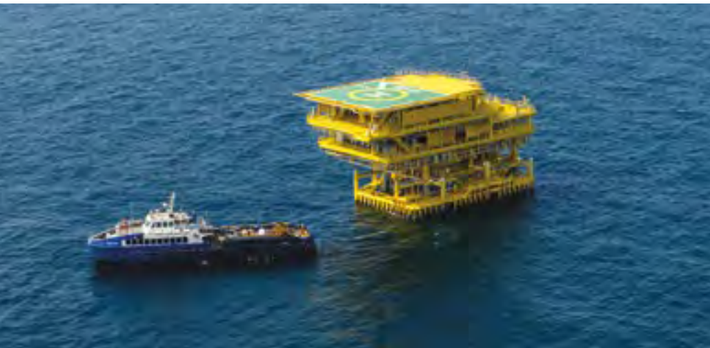
▲ Newly-installed wellhead platform Arabian Gulf
