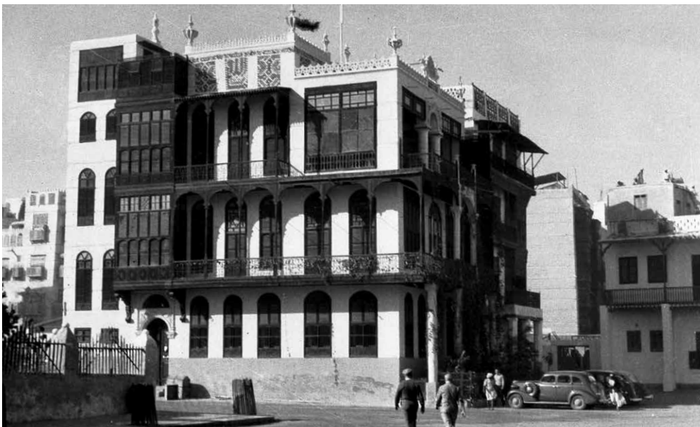
In late 1934, Lenahan moved Casoc's Jiddah office to more modern quarters near the city's Medinah Gate. The new building, which became known as the Bait al-Amerikani, had an interior designed to his specifications.
