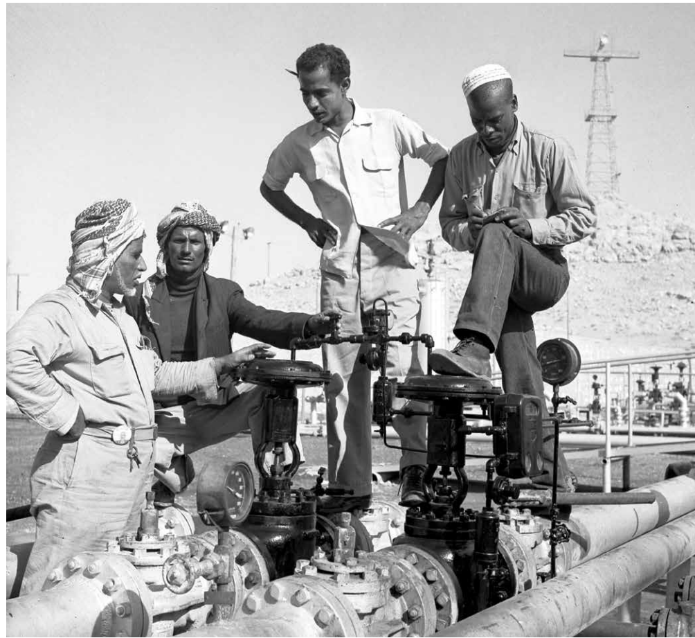
Saad bin 'Agil provides instruction to Ahmad bin Saad, Muhammad bin Abdulaziz, and Yagoob bin Yousuf, left to right, in 1954. Operating a back pressure gas regulator was only one of many tasks that potential GOSP operators had to master.
