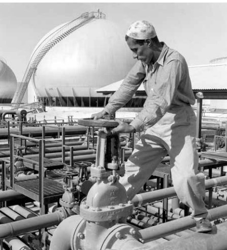
'Id bin Ahmad opens a gasoline-blending discharge valve at the Ras Tanura blending and transfer pump house in 1956, a year in which the refinery processed more than 70 million barrels of oil, nearly double the amount of 1950.
