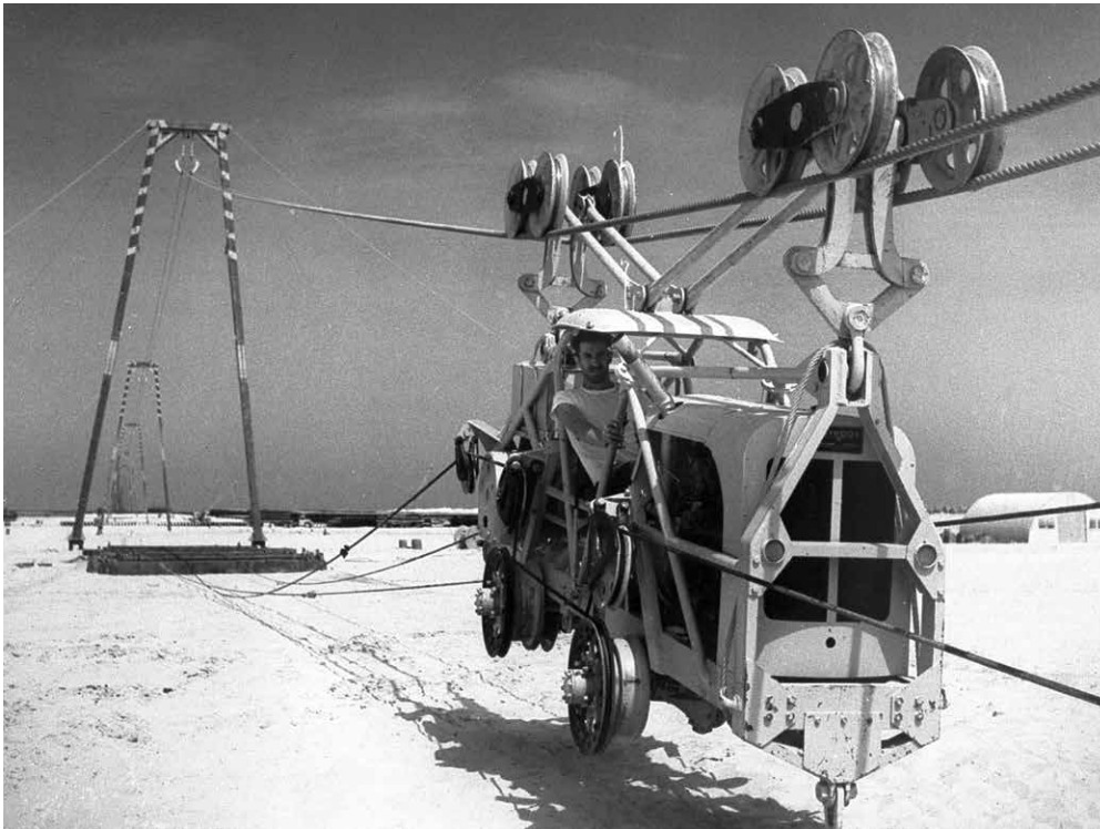
An operator tests the Sky Hook at the port of Ras al-Mish’ab on April 4, 1948, before it began carrying Tapline pipe sections from ship to shore. The overhead cables, which stretched nearly five kilometers, were modeled on equipment used in the logging industry.
