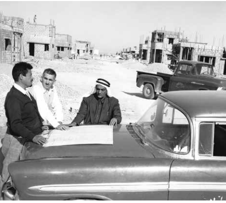
Surrounded by the half-completed homes of the Madinat-Abqaiq development, Ralph Tufley, from Aramco's Home Ownership Program, meets with contractors Muhammad Al-Khatib and Hamad Abu Nahyah to discuss construction progress in 1958.
