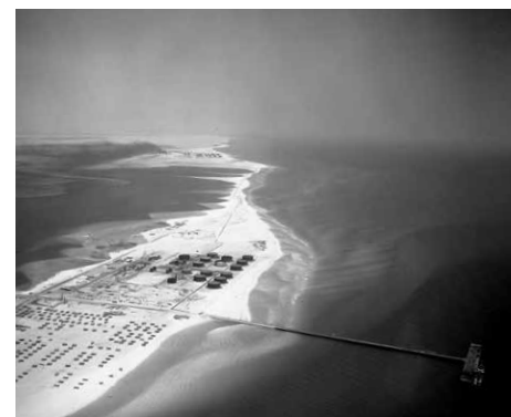
Shown in the mid-1940s, the Ras Tanura Refinery complex spanned the entire width of a narrow sand spit. Rows of tanks stored oil for export tankers calling at the terminal.
