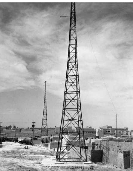
Radio towers dominate the skyline of Riyadh in 1950. While the government of Saudi Arabia worked to modernize Riyadh and other cities, it relied very much on Aramco in the development of infrastructure in the Eastern Province.
