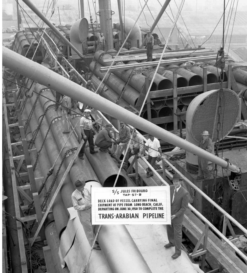
The last shipment of steel pipe for Tapline is loaded at Long Beach, California, in June 1950.
