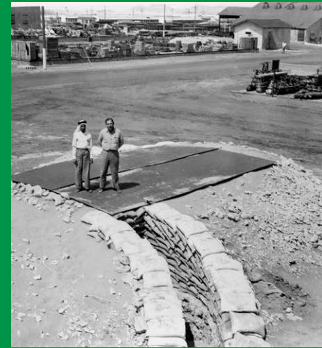
After an Italian war plane mistakenly bombed Dhahran in October 1940, Casoc built 25 air raid shelters in Dhahran and Ras Tanura. The shelters, such as this one in Dhahran, featured roofs of steel plate over layers of sandbags.
