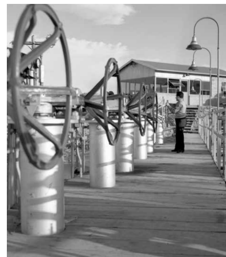
A worker adjusts a valve at Tapline’s Sidon, Lebanon, terminal where the first tanker arrived December 2, 1950. In 1951, its first full year of operations, the Sidon terminal received 14.2 million barrels of oil from Tapline. Seven years later, the figure had risen to more than 135 million barrels.
