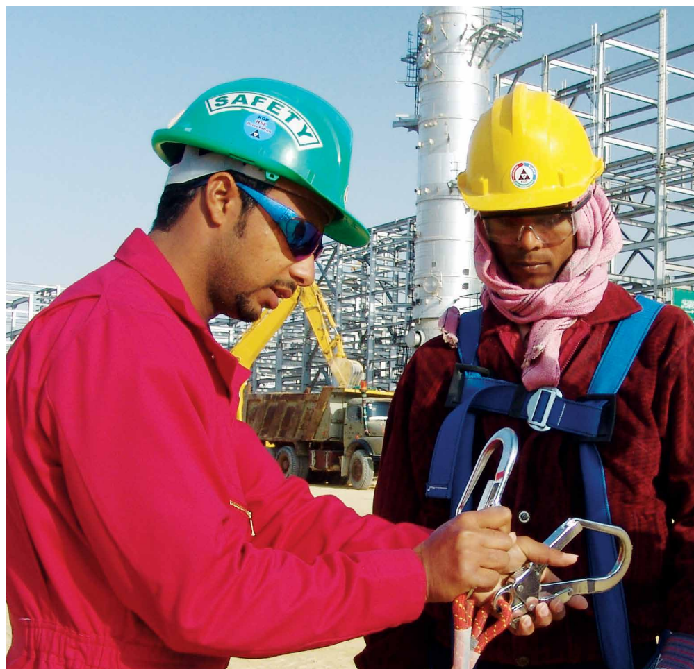
Fawaz Hassan, left, a safety officer with a contractor company on the Khursaniyah Gas Plant project, discusses proper safety harness rigging with a fellow employee early in 2007. Hassan was one of thousands of young Saudis trained to take on important construction jobs essential for the success of the long list of Aramco projects under way in the mid- to late 2000s.
