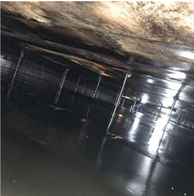
Figure 3: Inside T-2041 after completing the process
