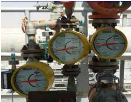
*The implementation of wireless purge flow meters reduced gas emissions by cutting fuel gas consumption by 11%.*
